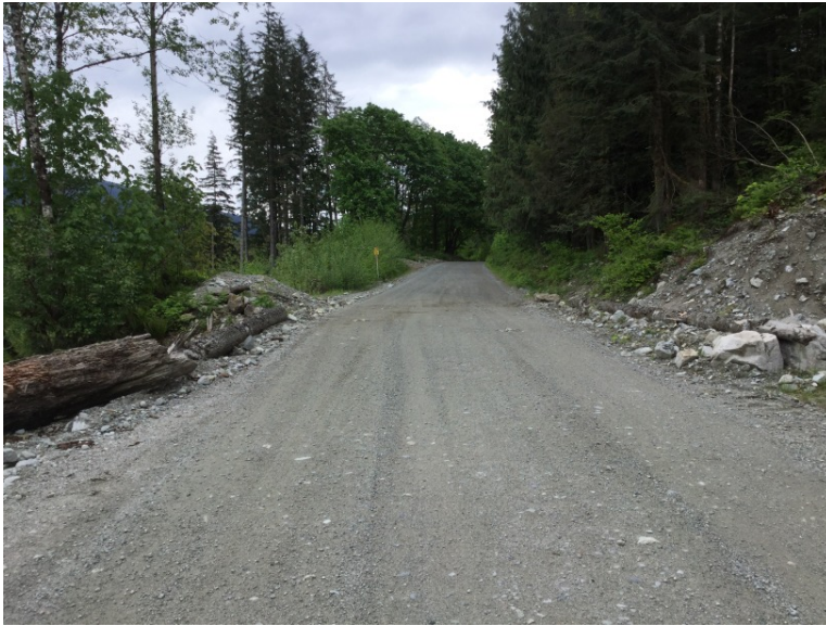
Approach from Left Bank when facing downstream
