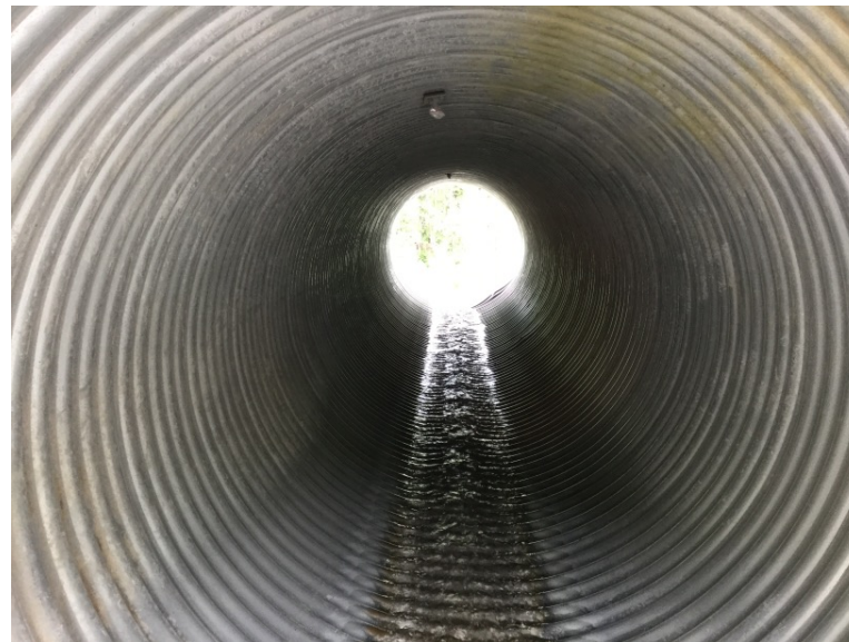
Looking through from inlet
